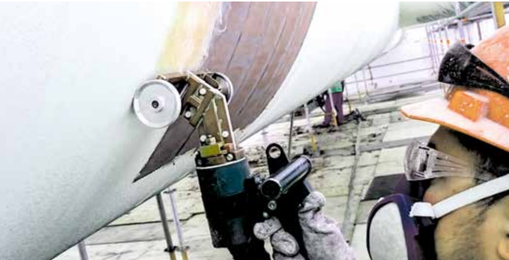
The Coating Removal System effectively removes industrial coatings of almost any thickness.
