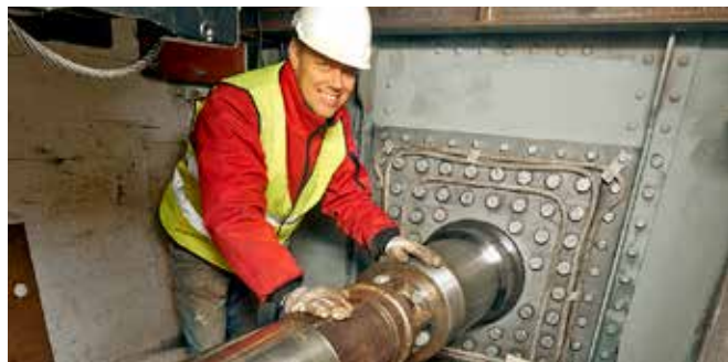
Induction shrink-fitting the shafts of an old bridge.
