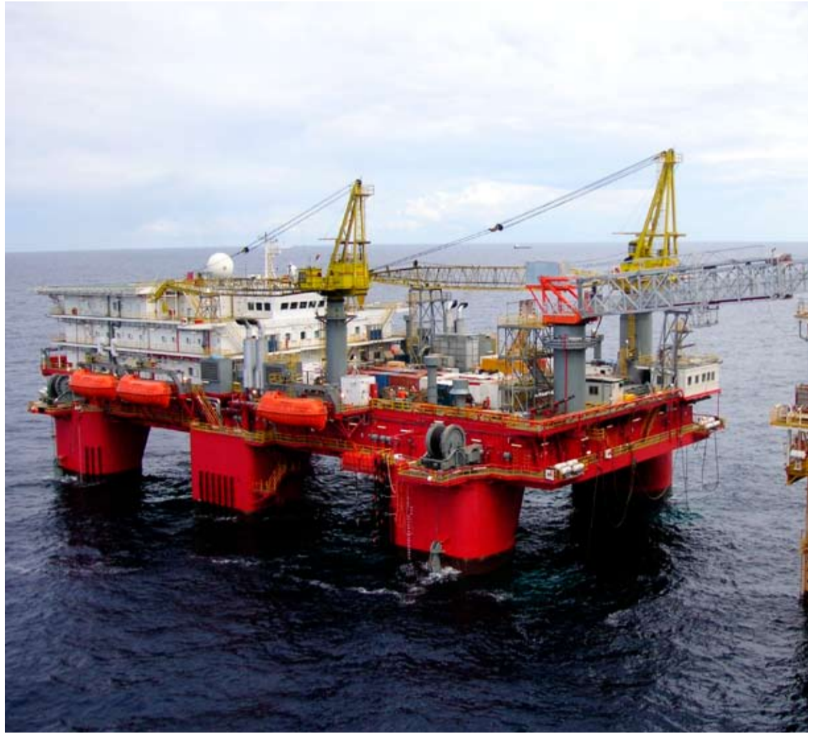
Prosafe’s ‘Safe Concordia’ accommodation and service platform. Flameless induction heating was used to pre-heat a section of crane tower that also serves as a control room bulkhead. “© Prosafe”
