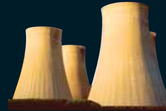
Brazing of copper parts in generators. Shrink- fitting. Bolt expansion. Pre/post heating and brazing for high-pressure turbines.
