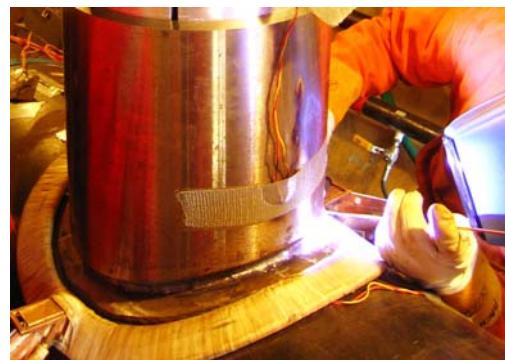
Welding the branch (coils 2 and 3 not visible)
