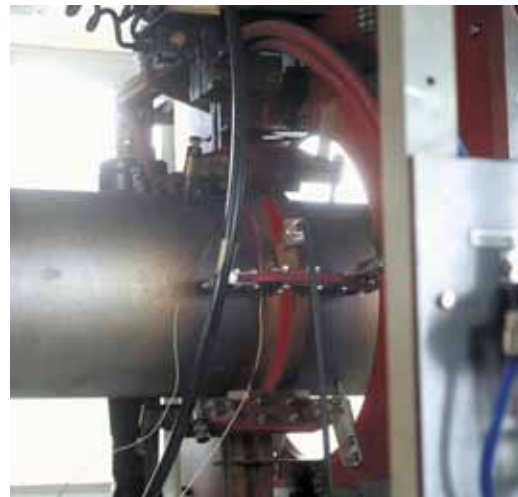
High-throughput post-weld induction heat treatment of offshore pipe.
