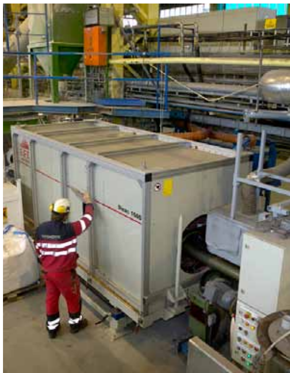
An example of induction pre-heating: the pipe is being heated prior to receiving an anti-corrosive coating.
